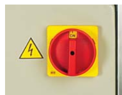
FVG - Main switch for emergency stop
